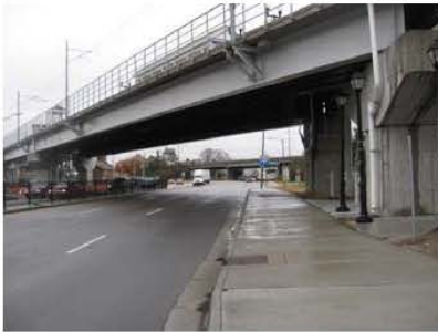
Brambleton between Park and I-264, looking east (2014)
