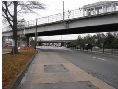
Brambleton between Park and I-264, looking east (2014)
